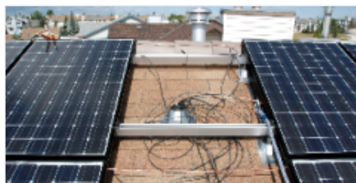
Installing the panels.
