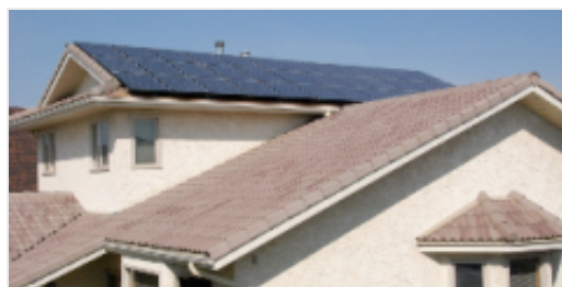
At peak, the 36 module, 200 W Sanyo system is expected to generate 6-7 kW on average.
