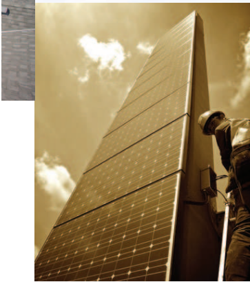
Ralph Klein Legacy Park, 2.2 kW grid-tied solar electric system
