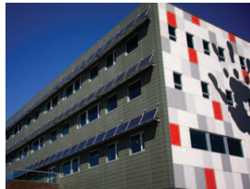
Child Development Centre, University of Calgary, 43.4 kW grid-tied solar electric system (largest system in Alberta)
